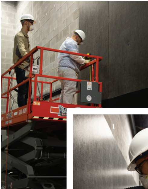
Media production staff install soundproof paneling in our new studios.
