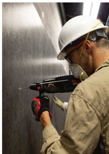
Media production staff install soundproof paneling in our new studios.
